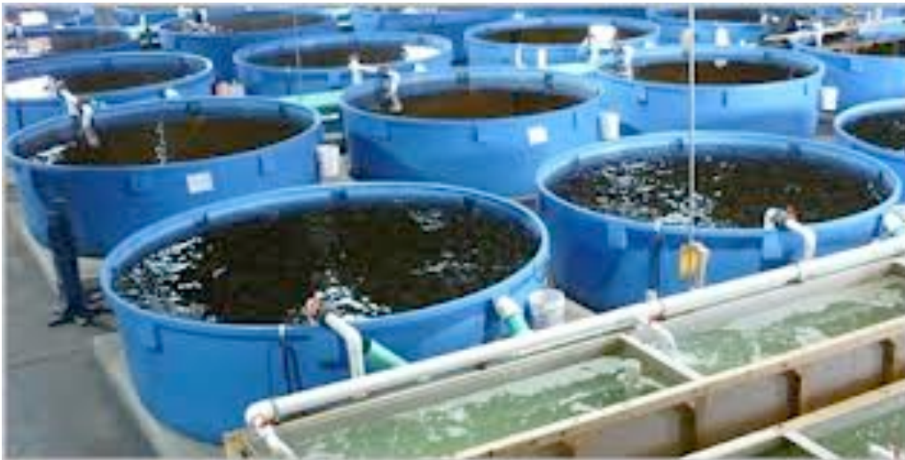
Figure 2: Closed containment system grow-out tanks
