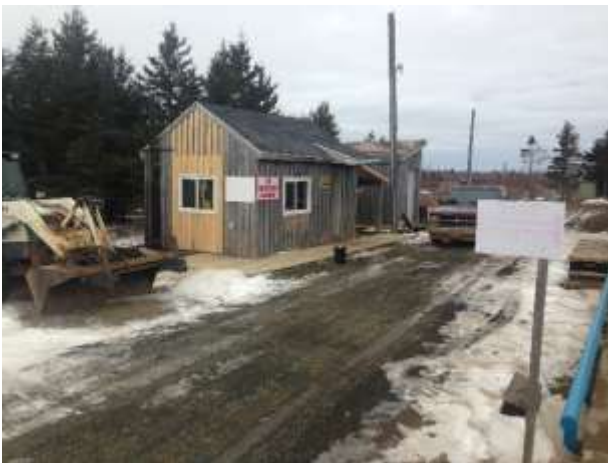
Photo 18: On site office and scale house.
