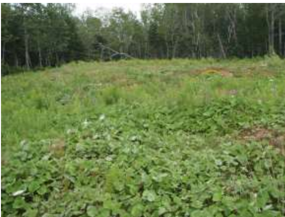
Photo 14: Covered and vegetated Phase 1 asbestos disposal cell.
